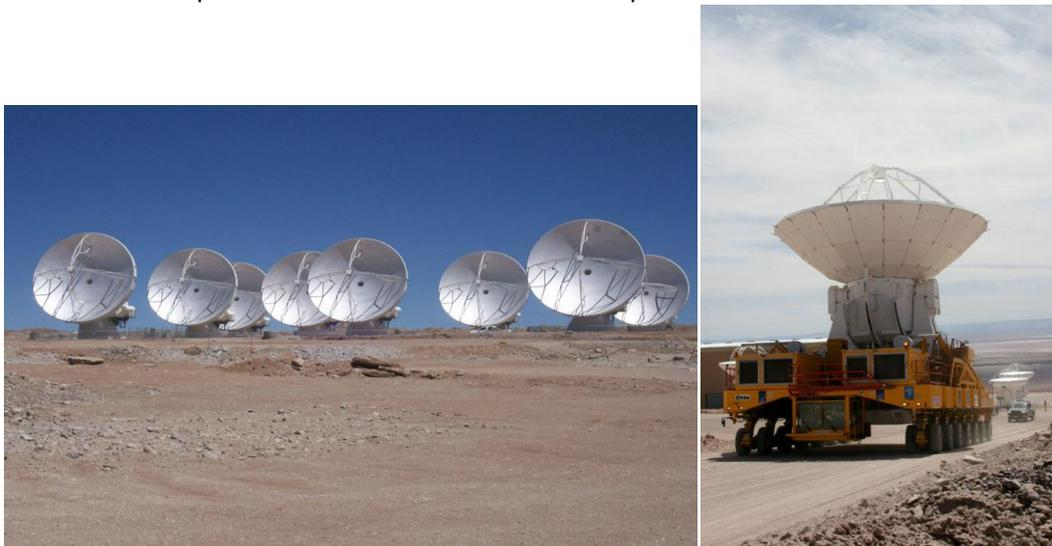
Figure 66. The ALMA array with eight 12-m antennas (left), and an antenna being transported to the AOS (right).
