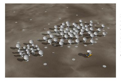
Figure 7: Artists conception of the ALMA 12-m Array in its compact configuration, with the ACA toward the left, and the transporter in the lower right. A few unoccupied pads can be seen, to which antennas of the 12-m Array can be moved by the transporter as the array is being reconfigured. At its most extended configuration, antennas in the 12-m array will be up to 16 km apart (see Figure 8). © ALMA (ESO/NAOI/NRAO)
