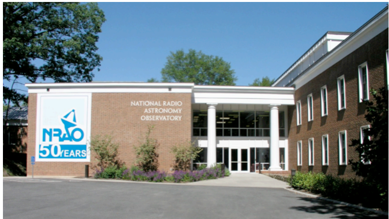
Figure 1: NRAO Headquarters and location of the NAASC
