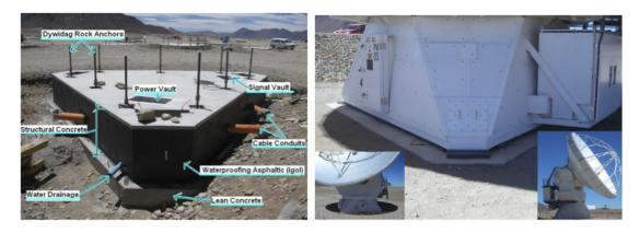
Figure A.2: Structure of an antenna pad (actual pad at the OSF) (left) and detail of antenna anchored to a pad (right).
