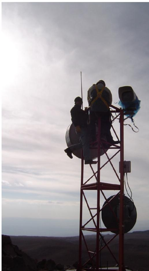
*IT and contractors installing the first communication link in Chajnantor (Cerro Chico) pointing to AOS-TB*
