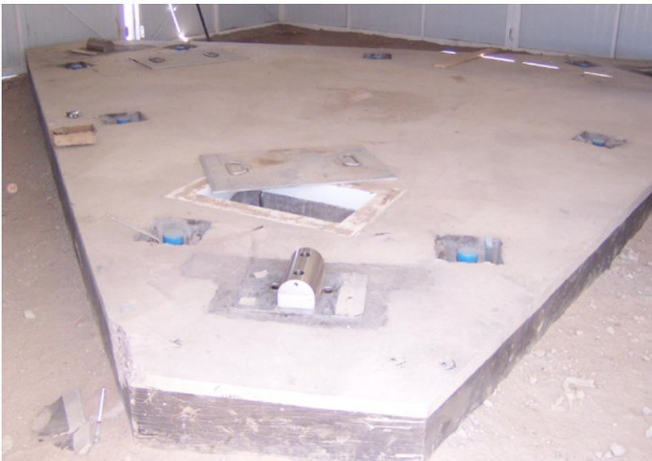
*Photo of an Atacama Compact Array (ACA) antenna foundation showing the three inserts that are used to accurately position the antenna, and the connection devices (so-called "vaults") for signal transmission to command the antenna and to transmit signals from the receivers to the correlator, and power. The correlators for the ALMA interferometer array and the ACA are located in the AOS Technical Building. After correlation, the data are transmitted to the OSF.*
