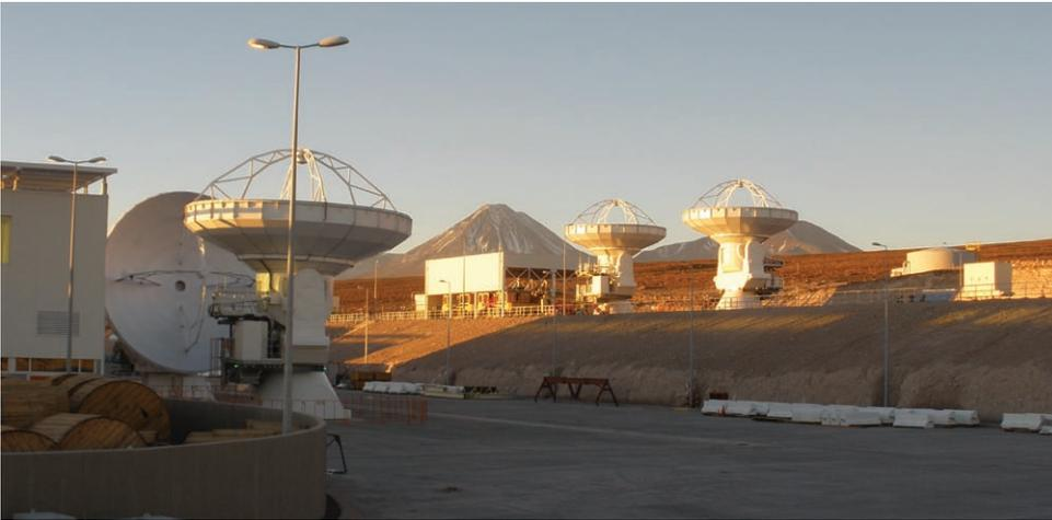
Antennas are moved to the AOS after being conditionally accepted at the contractor's site and moved to the OSF. Each antenna is outfitted with electronics and put through exhaustive tests at the OSF by the Assembly, Integration and Verification (AIV) team. So far, twelve antennas have been conditionally accepted by the Project and have entered into this process. After outfitting and initial tests, the antennas at the OSF are
