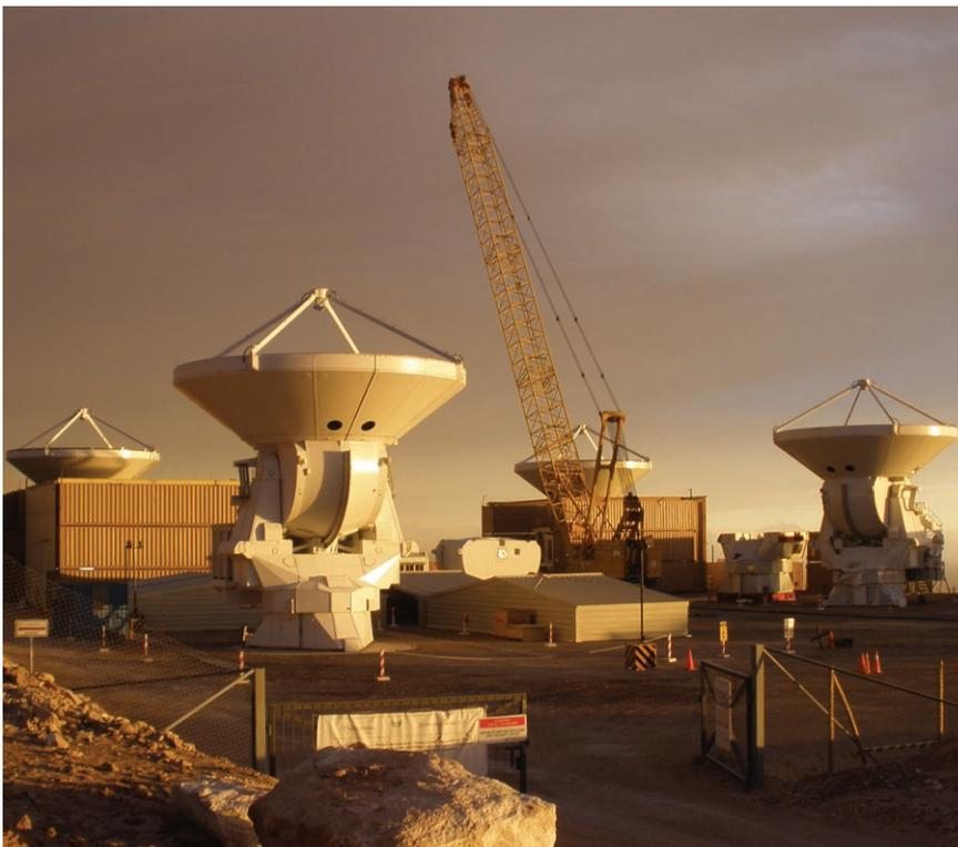
Significant progress has been achieved at the European Antennas assembly site as well, where one antenna is ongoing acceptance testing while five others are in different stages of assembly.
